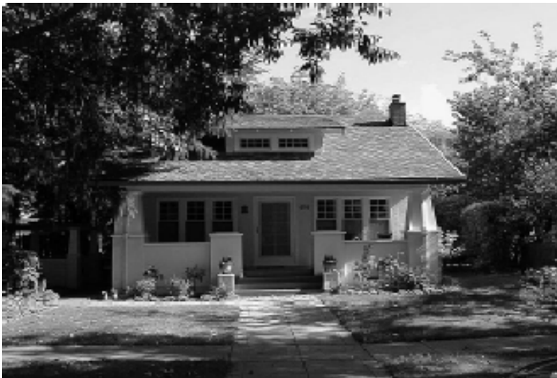
A bungalow with a full-width inset porch
